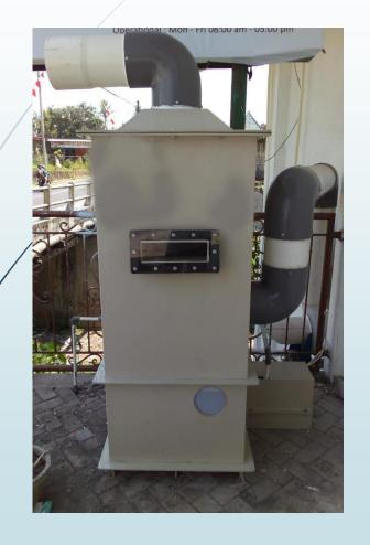
**A Wet Scrubber** is an air pollution control device that removes PM and acid gases from waste gas streams of stationary point sources.
